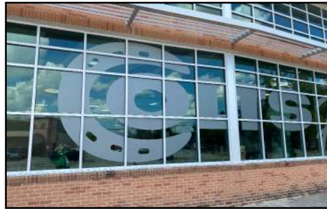
Etched windows on Cafeteria facing Park Row
